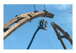
Left: Crew from Dane Construction works with two crane operators to close the gap between the two arms of the wooden arch for City Walk's pedestrian bridge over NC 127.
