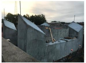
Photo cutline: The abutment for the east end of the pedestrian bridge over NC 127 is complete. Girders spanning the roadway will rest on the abutment's lower ledge while the walking service will be at the upper level. The four slanted pillars are decorative. The bridge should be complete in September.
